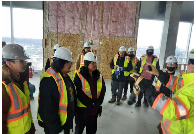
Students spent the day listening and learning about all the different trades that are involved in a single structure.
